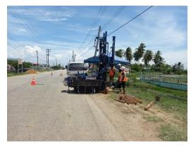
With the Government of Guyana's plans to rehabilitate the New Amsterdam to Moleson Creek Road Corridor, CBA was contracted to provide soil testing at each structure location along the road way from Brighton to Moleson Creek. This project include subsurface investigation via cone penetration testing (CPT) and standard penetration testing (SPT) at 50 structure locations along the road corridor.
