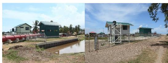
The Nootenzuil Drainage Pump Station (E.C.D, Guyana) consists of a single 120 cusec pump module. CBA was conracted to design and supervise the construction of the pump station, sheet pile bulkhead, access road and ancillary works. Similar pumping stations were designed and supervised by CBA at Hampton Court (Essequibo), Devonshire Castle (Essequibo) and Hope (E.C.D).
