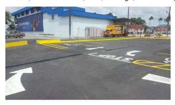
CBA was contracted to provide design and supervision services for a *Parking Lot Facility to the DSL Supermarket at Great Diamond*, E.B.D (Guyana). The parking lot requirements included a flexible pavement with asphaltic concrete wearing surface, entrance
