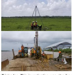
provided geotechnical services for Tristar Inc. This investigation was also for a shorebase facility and included three (3) 35m deep boreholes.
