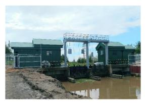
CBA was contracted by the National Drainage and Irrigation Authority (NDIA) to undertake supervision services for the rehabilitation of the drainage pumps at Three Friends, Essequibo Coast (Guyana). The dual 150 cusec pumping station was redesigned during the supervision stage and delivered within the contract period by the consulting team.
