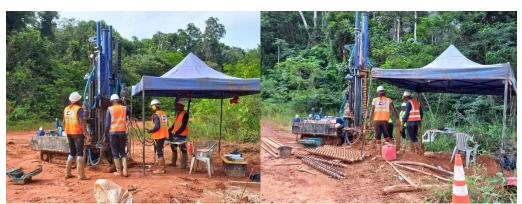
**ETK INC.:** C.B. & Associates Inc. provided geotechnical services for the bridge foundation designs for the upgrade of the South Access Road (SAR), Puruni, Region No.7. Cone penetration testing (CPT) and standard penetration testing (SPT) via continuous auger drilling were conducted.
